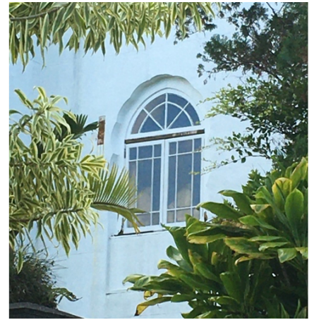
Mar-Original Windows Installed
