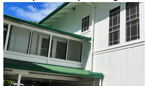
Dec-"Bridge" Windows SOON!
