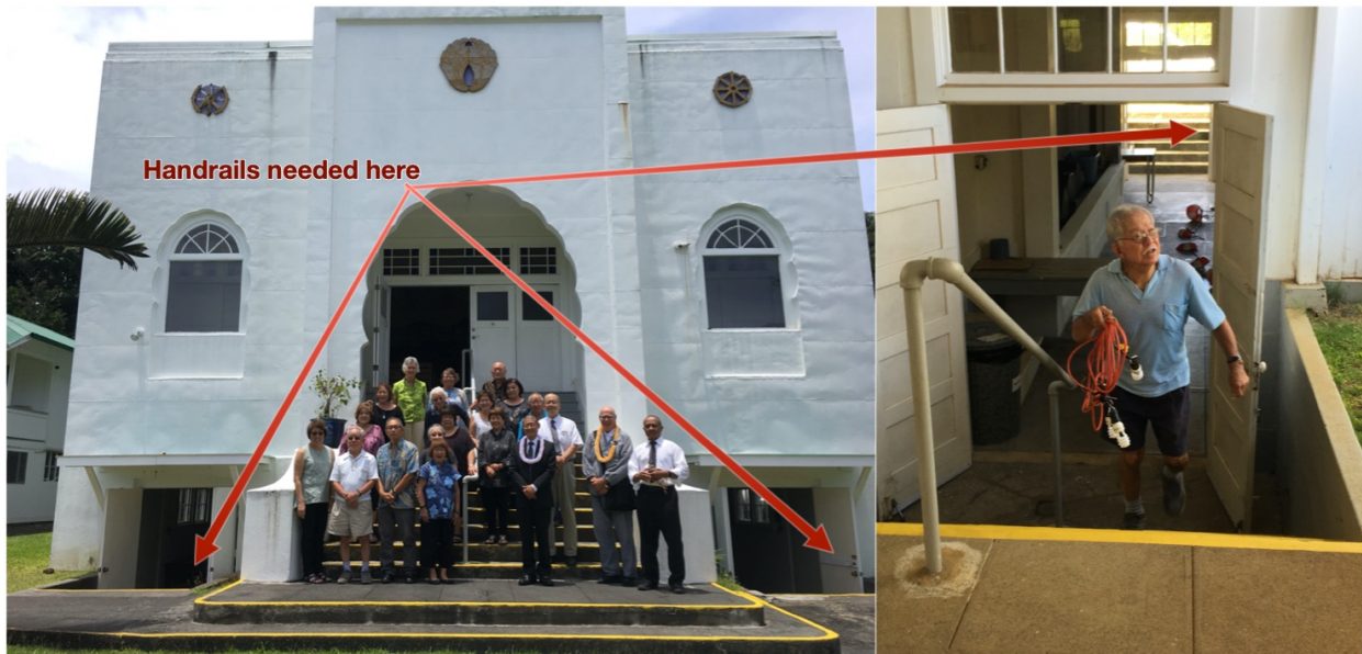
2019 Fujinkai Convention gathering shows two of the stairwells in need of handrails. The 2019 photo of Clyde Chinen setting up for Obon shows the 3rd staircase requiring handrails and the only staircase into the Social Hall that has handrails.
