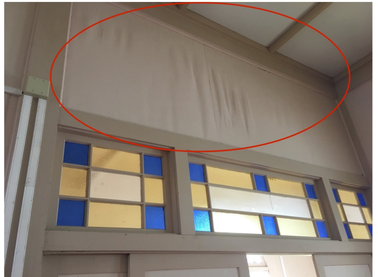
We will repair termite damage.
