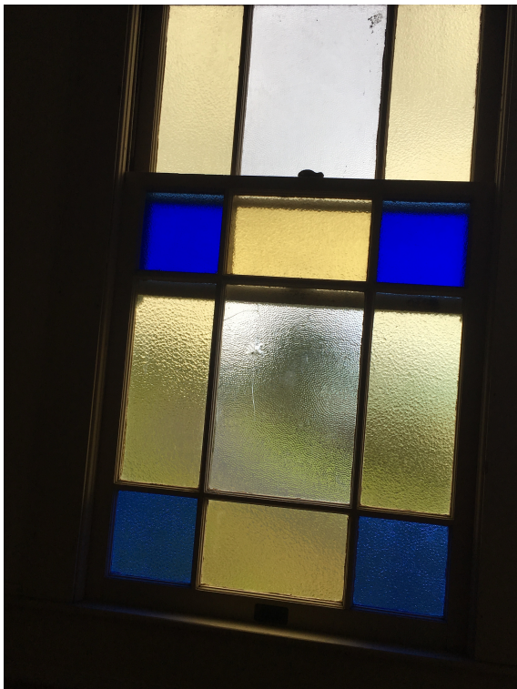
We will replace broken panes & make sure the windows function well.
